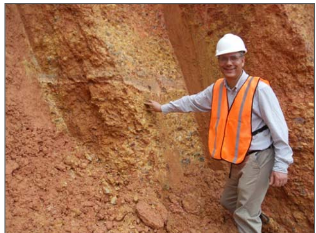
Figure 1. Saprolite Soils Maintain the Intact Rock Structure – A Saprolite Excavation Profile at a Site in Panama
