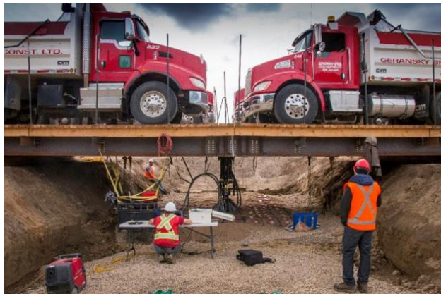
Figure 1: Large scale plate load testing during the summer of 2019.
