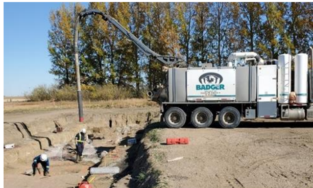
Figure 4: Vacuum truck used to exhume interface surfaces in 2021.
