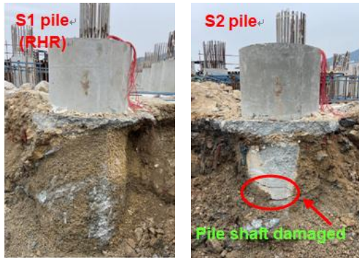
Figure 9. Test results of pile integrity
