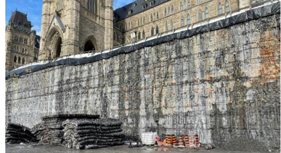
Figure 2: PWC partial north excavation face (Peace Tower foundation middle left).
